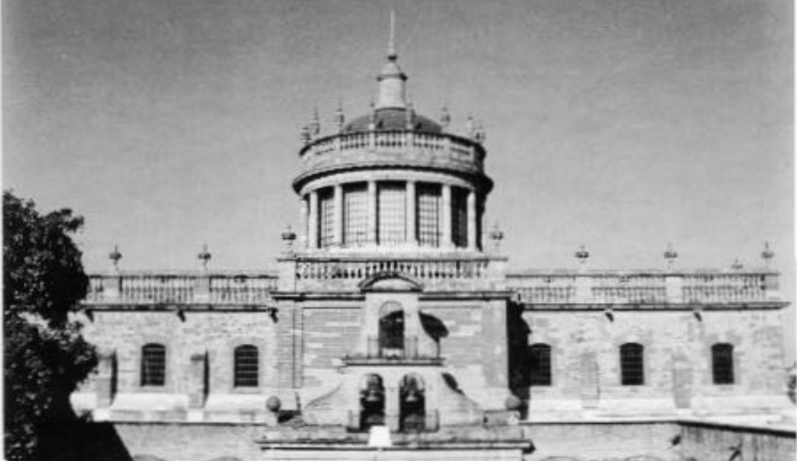
Guadalajara : Façade de la chapelle / Main facade of the Chapel
