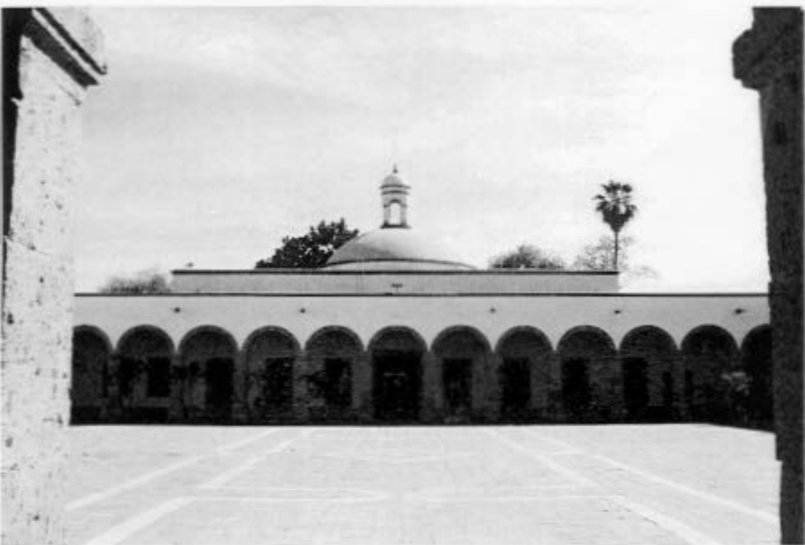
Guadalajara : Façade de la cuisine / Main facade of the kitchen
