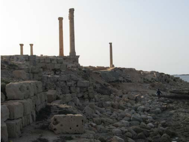
Figure 3 Temple of Isis, erosion of structures caused by the sea
