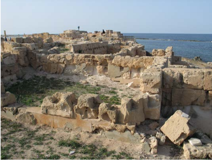
Figure 5 Sabratha Deterioration of sandstone constructions
