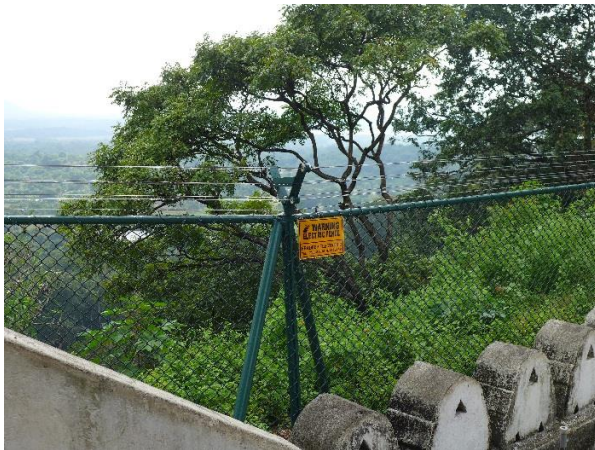
Figure 9 Electric Fence to Protect Against Monkeys Entering
