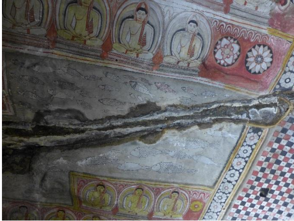
Figure 17 Water Leaking from the Ceiling
