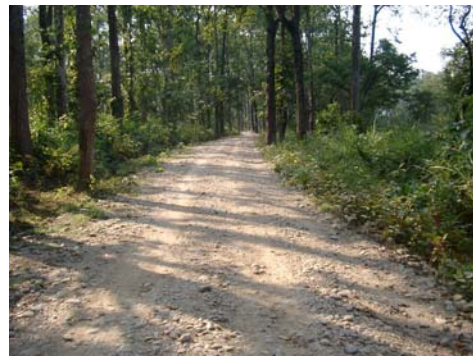
Fig. 4 Link road connecting Kasra Bridge to the public right of way
