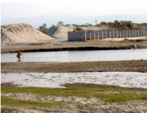
Fig. 11 Causeway under construction over the Reu River
