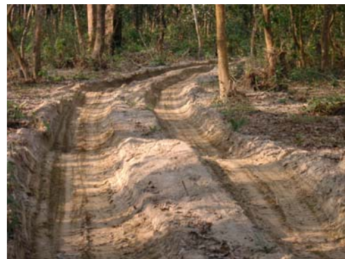
Fig. 12 Condition of existing road used by vehicles crossing the Rapti River to connect to right of way
