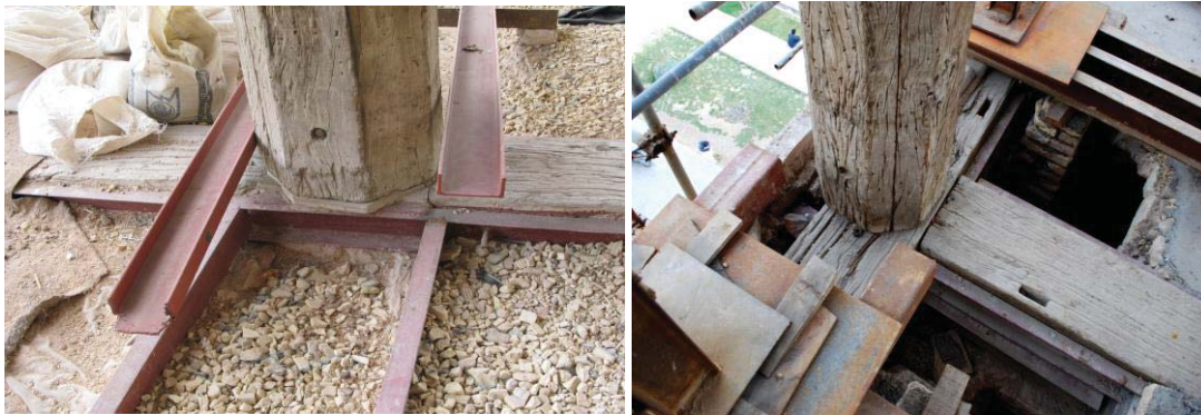
Figure 3. Stabilization of the porch
