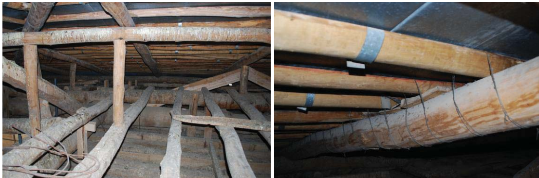
Figure 4. Stabilization of the buttresses
