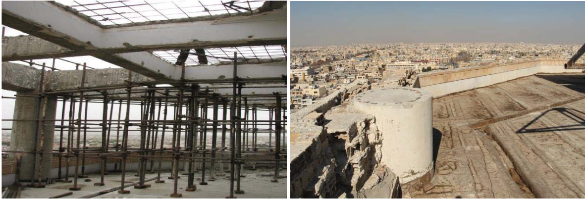
Figure 2. Demolition of the upper stories of Jahan nama building
