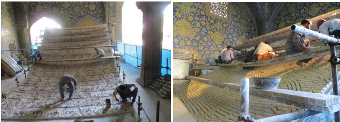
Figure 6. Stabilization of the dome's decorations
