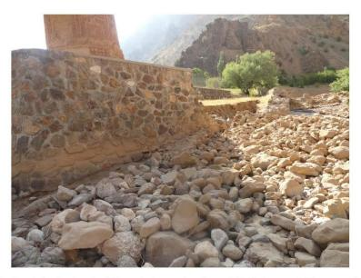
Once again floods in the Jam Rud River during spring time of 2012 damaged 30 meter of retaining wall as will a lot of stones brought by floods on the bed of river which needed for cleaning.
