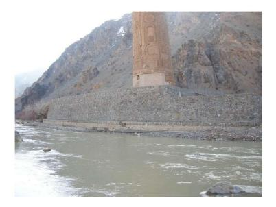
New retaining wall on the bank of Hari Rud River has been built on 2007 total length 55 meter with the height of 8 meter and wide of 2 meter. The retaining walls on Hari rud are still in good condition no cracks, no cavities, no distortions.
