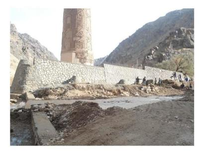
By the financial support of MoIC and UNESCO office a strong retaining wall with the length of 45 meter and height of 4.5 meter has been constructed on the bank of Jam Rud River on 2014. As will flood breakers in several points of Jam Rud River have been implemented to reduce the power of the floods.
