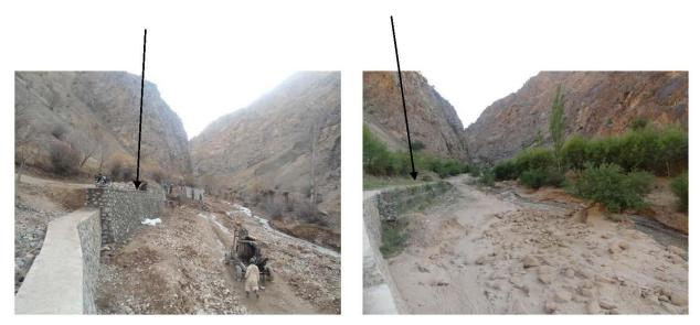
In addition in the rout of Jam valley the gabion wall (Jam Rud River) which was in bad condition has been removed and new retaining wall has been constructed with length of 50 meter and high of 4.5 meter. 2014
