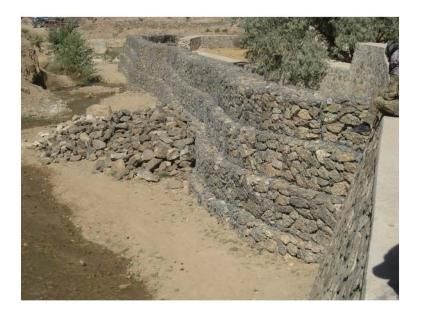
For the safeguarding of the minaret against the seasonal floods, a temporary retaining gabion wall has been constructed in the bank of Jam Rud River with the financial help of US Military Founding. Since the constructed gabion wall is considered as temporary solution, and the width of the Jam Rud River has been narrowed, this gabion wall completely removed on September 2014.
