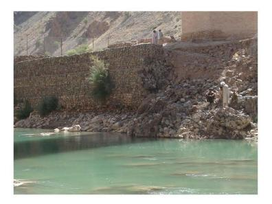
Gabion wall on the bank of Hari Rud river total length 43 meter with the height of 5.5 meter has been built on 2000 a part of the wall destroyed due to heavy floods on 2007.
