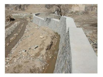
Retaining walls on the bank of Jam Rud River has been built on 2007-2009 total length 110 meter with the height of 4 meter and foundation wide of 2 meter.
