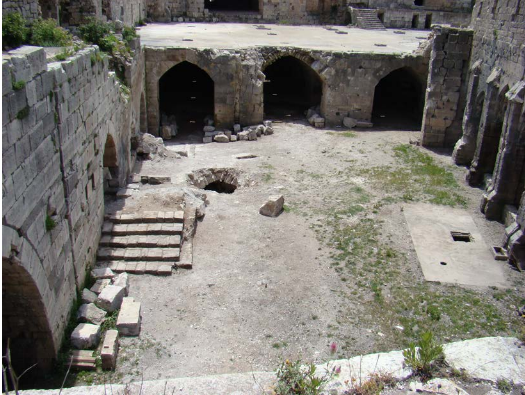
The interior courtyard in Krac des chevaliers (After) - © DGAM 2014
