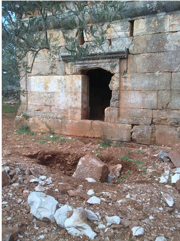
Illegal excavations at al – Bara, Zawia Mountain, Idlib Countryside - © DGAM 2014
