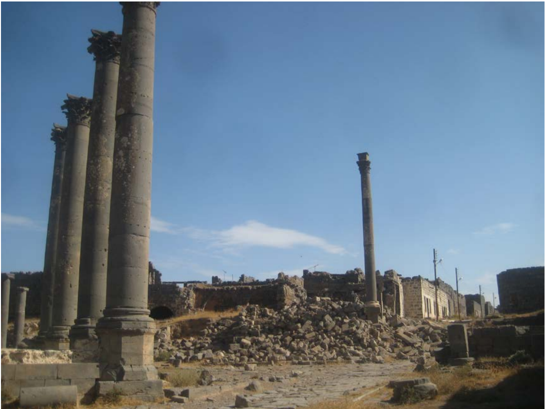
Severe damage to Kalybe, "Cradle Of The King's Daughter" in Bosra © DGAM 2014
