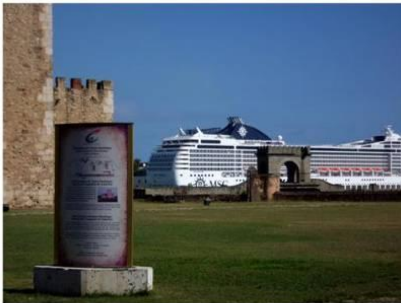
Impact of big cruise ships anchored immediately in front of the Fortress.
