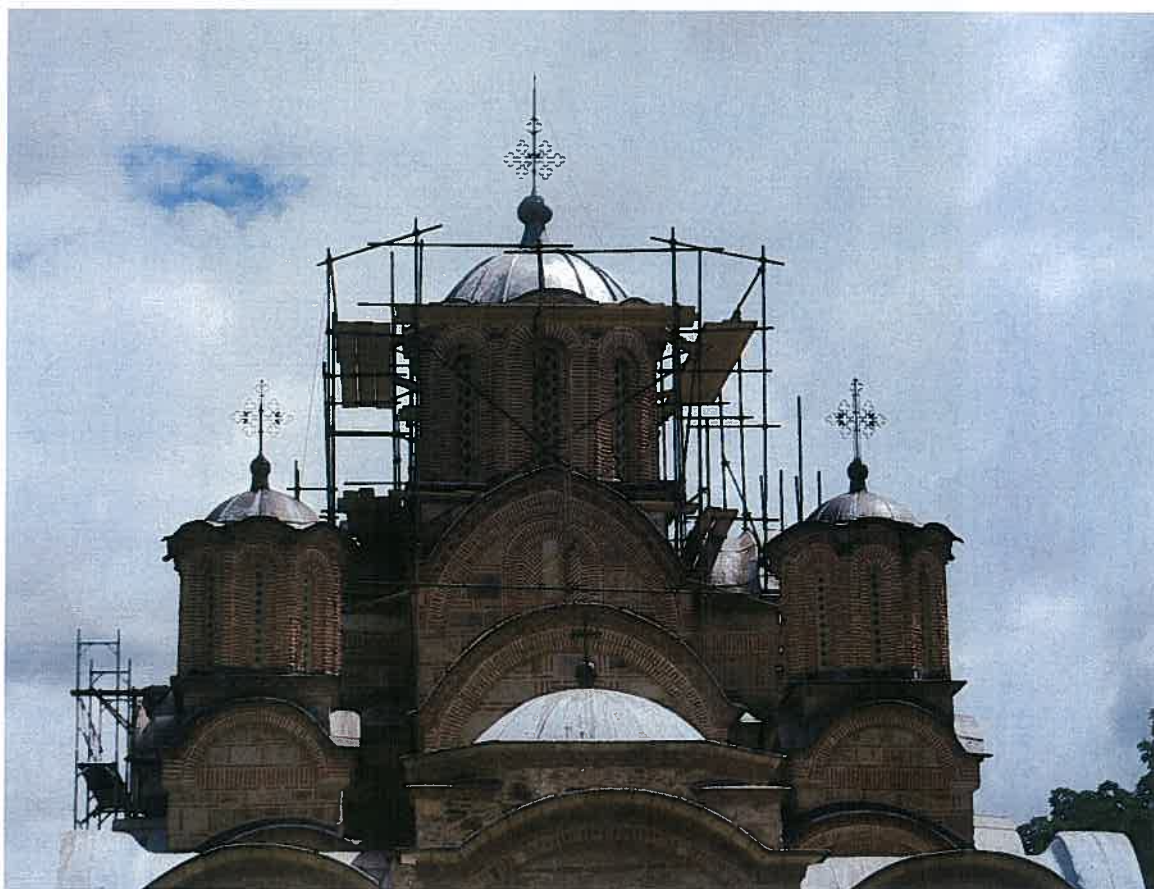
Monastery church during works
