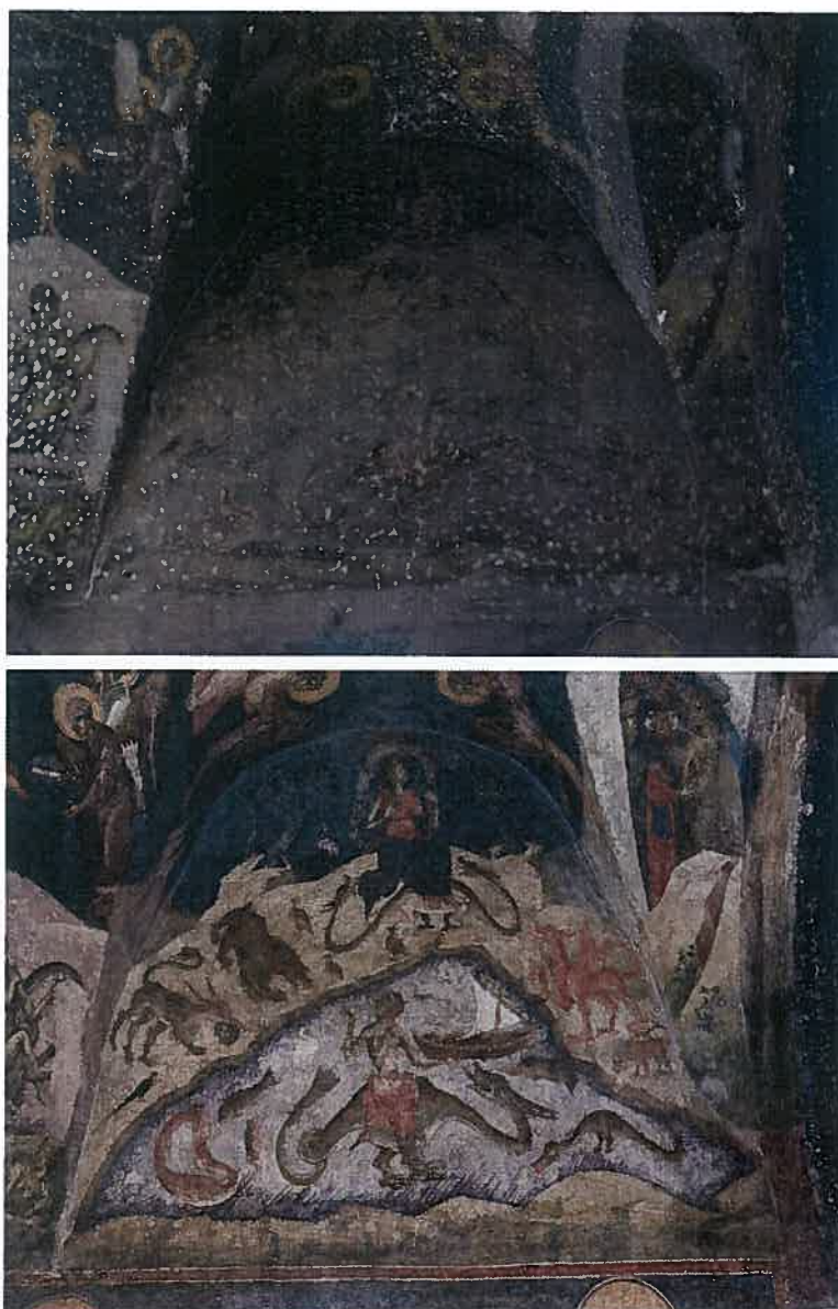
Detail of wall paintings before and after the conservation works
