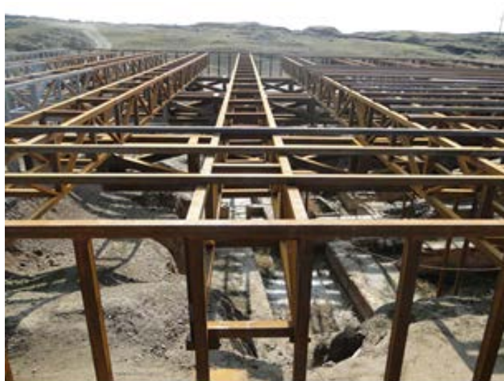
FIG.3 Protective shelter during the work (Source; Department of antiquities of Sherqat,2013)
