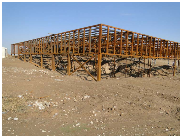
FIG.4 Protective shelter from south-west corner (Source; Department of antiquities of Sherqat,2013)
