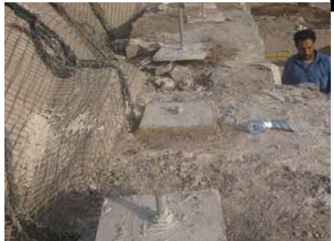
*Figure 2: Strengthening the join between a pillar and an arch with Geogrid mesh and plastic (Teflon) plate.*
