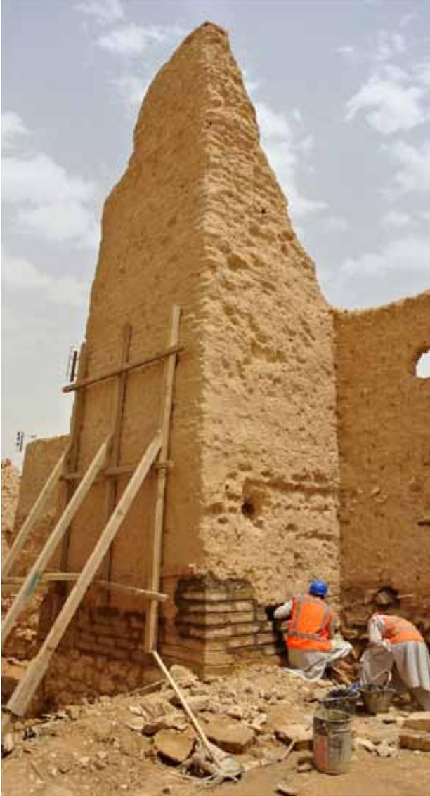
Figure 10: Pilot project: restoration works, columns restoration. © M. Bendakir
