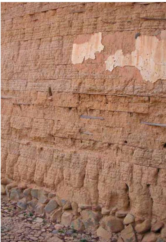
Figure 6: Features of *tulou* construction: a stone basement wall showing the bamboo wall bones. Source: [http://amuseum.cdstm.cn/AMuseum/hakla/image/jianzhuzhijianzhu\\_082\\_1.jpg](http://amuseum.cdstm.cn/AMuseum/hakla/image/jianzhuzhijianzhu_082_1.jpg)
