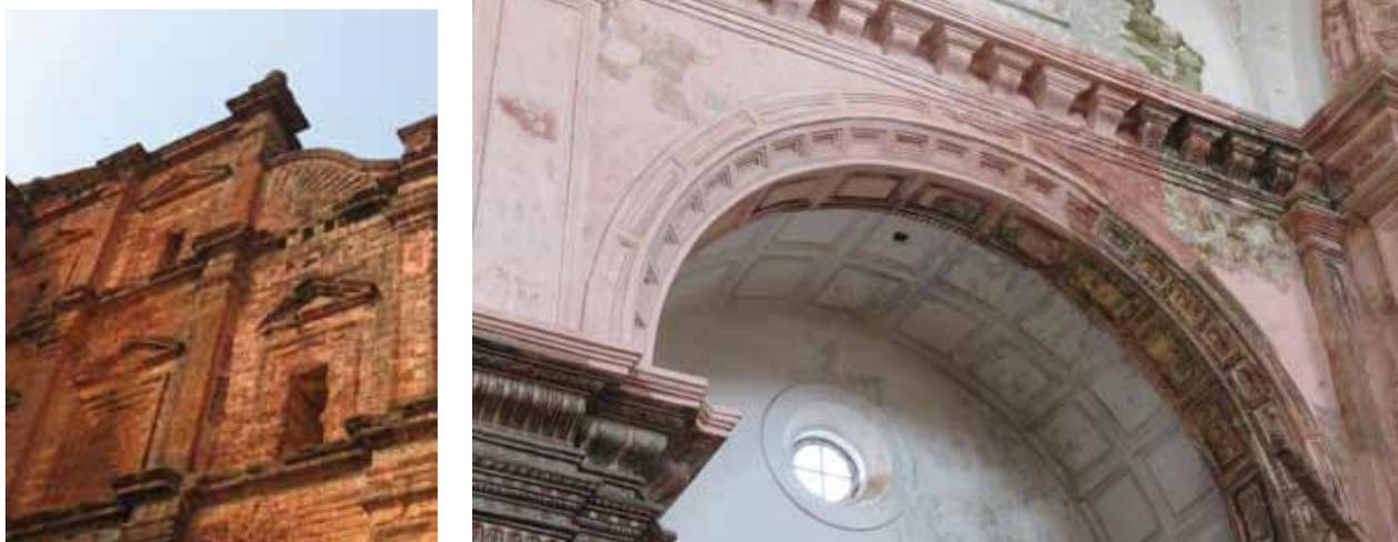
Figure 9: (L) Exposed laterite walls of the Basilica of Bom Jesus showing deterioration of the laterite blocks. (R) Water seepage from the roof affects the wall paintings inside the Church of St Francis of Assisi. © T. Sharma
