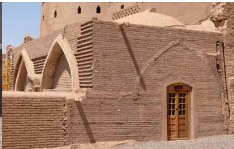
Figure 10: The stable after restoration, with arches and domes strengthened using fiberglass mesh.
