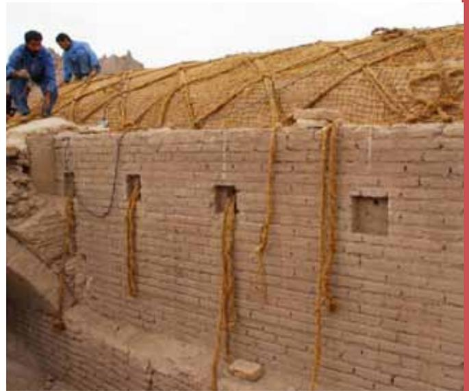
Figure 8: Strengthening an arched roof with rope and mesh made from palm fibre (SIS).
