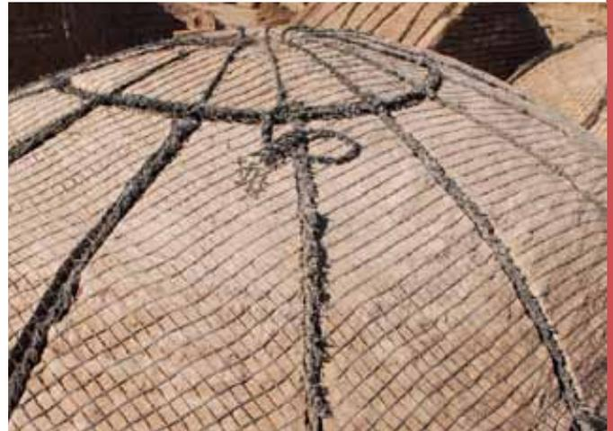
*Figure 1: A dome covered in Geogrid mesh.*
