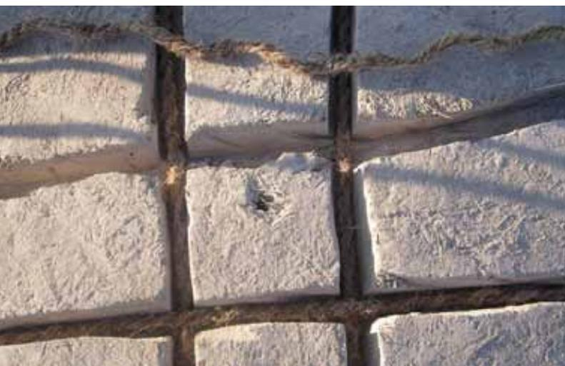
Figure 5: Detail of strengthening a dome by inserting rope made from palm fibre (SIS).
