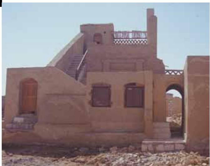
Figure 6: Eco-lodge prototype 'G' for Mr AbdAllah Schleifer, Tunness, Fayoum oasis. Egypt. 1992-93. The northern façade shows the entry tunneled corridor that acts as a suction wind shaft for all openings on it. This is in reflection as a little village scape within the small edifice calibrated in the fashion of the covered narrow streets of 'les Mzabes' of north Africa or the traditional oasis of the Egyptian deserts. © AHMAD HAMID ARCHITECTS
