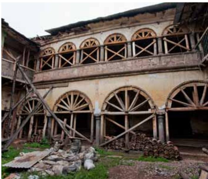
131 rooms arranged around two interior patios. Hotel El Comercio is constructed with rubble stone foundations, a fired brick masonry base course, adobe and fired brick masonry walls at the first floor, and *quincha* walls at the second and third floors (Fig. 9).
