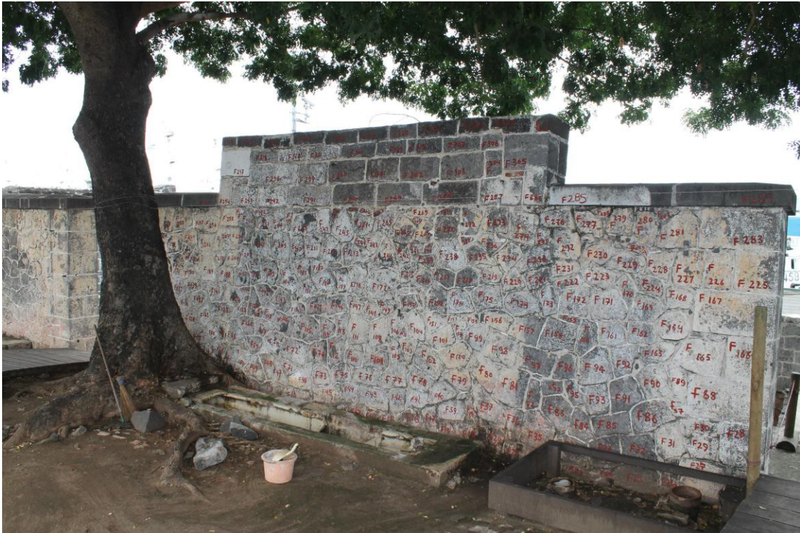
4 Photo: Inventory of the stones of the wall before a restoration work
