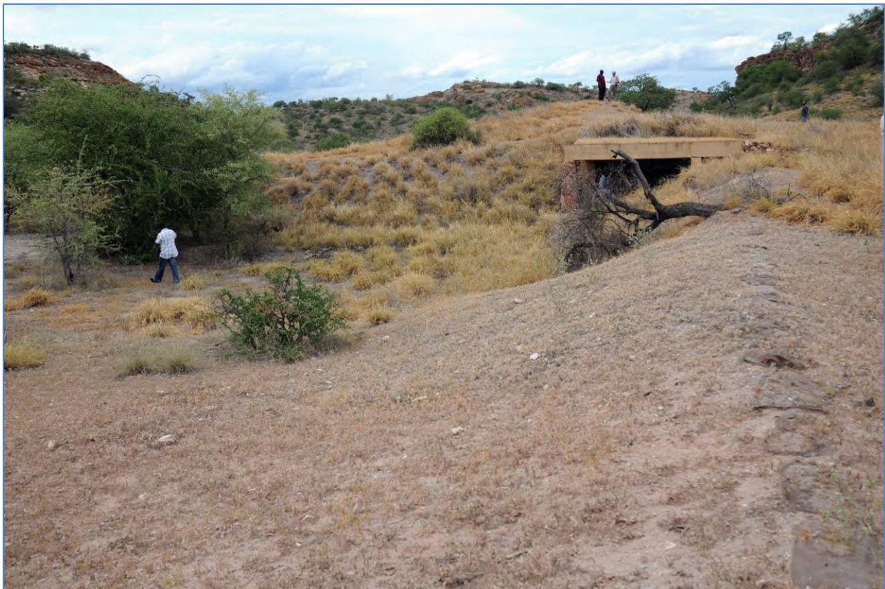
Figure 18. Earthworks and sandbags built to protect the K2 site from erosion. The system needs maintenance efforts, which can be seen from the exposed sandbags (visible on the left side of the picture). Photo: Dag Avango.
