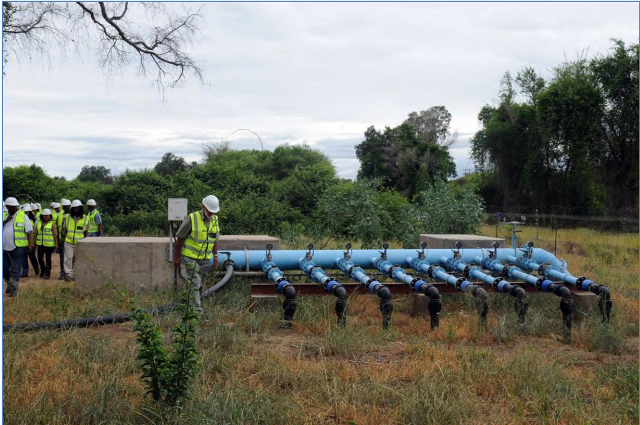
Figure 7. Water intake for the Vele colliery by Limpopo River. In the background the fence and barbed wire system along Limpopo River is visible. Photo: Dag Avango.
