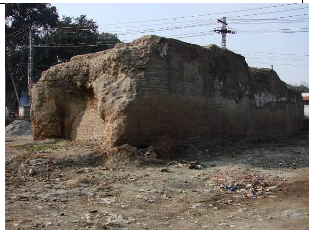
Picture box 2: Consolidation of the remains of hydraulic tanks at Shalamar Gardens
