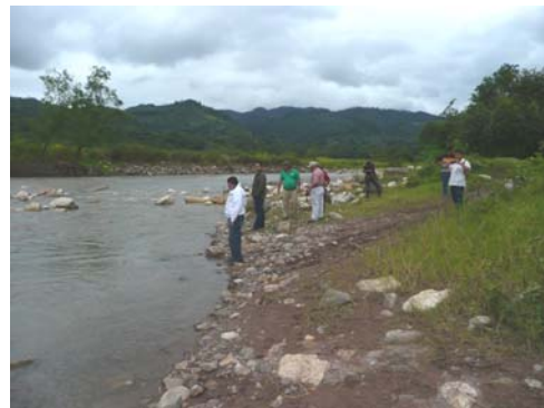
Image 11. Missing floodwalls along the river
