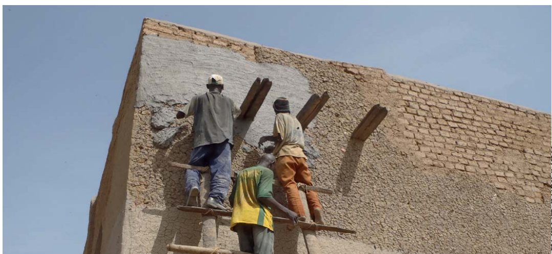
Rehabilitation of the Youth House in Djenné, October 2011
