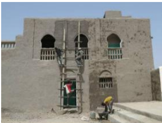
Final works on the main facade, Youth House, Djenné, October 2011
