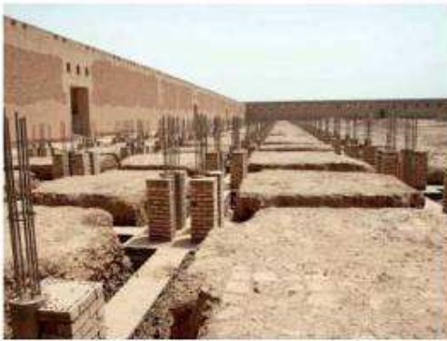
Foundation of the concrete columns reconstructed to roof the porticoes of the mosque.
