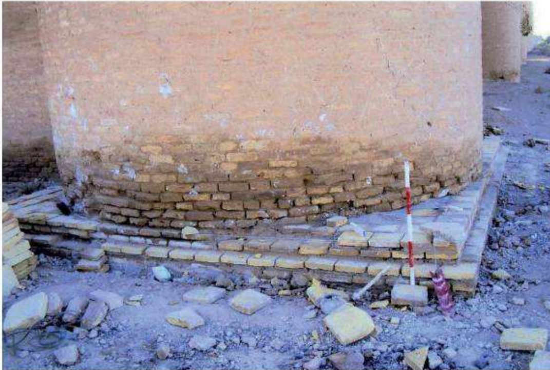
Treatment of basale erosion due to humidity and salts.
