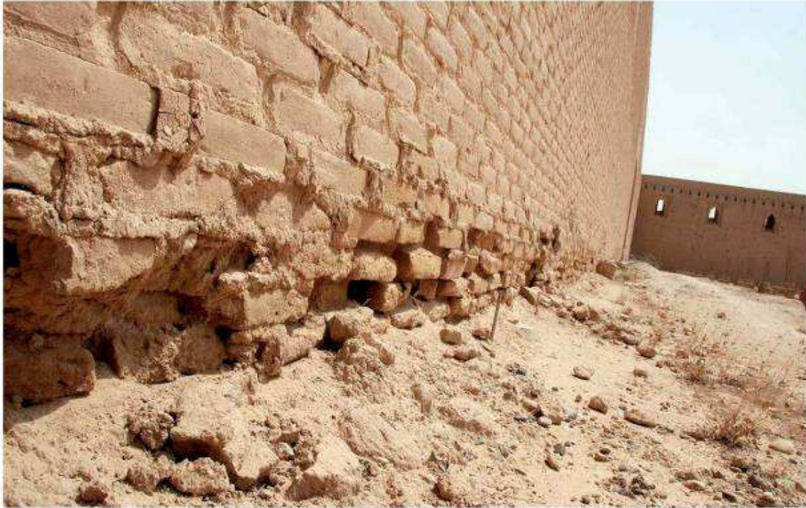
Humidity and salts pathologies, basal erosion of the Great Mosque walls.
