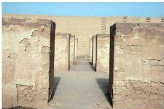
Erosion problems due to the incompatibility of materials, the reconstructed walls of the Al-Ma'shuq Palace.
