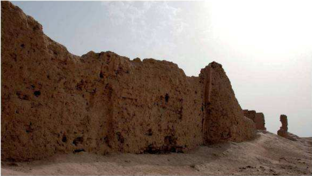
Erosion of the exposed outer wall of the mosque.
