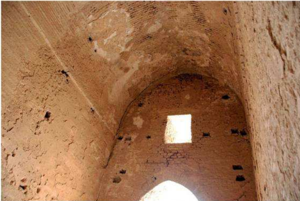
Humid pathologies of the vaulted gate of Bab al-'Amma, the Caliphal Palace.
