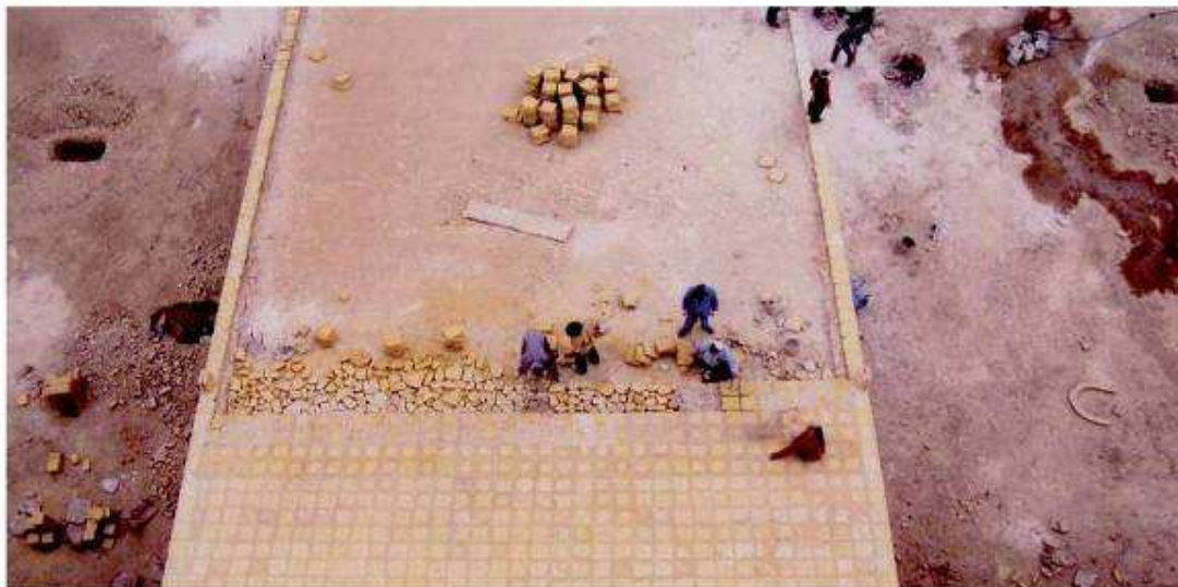
Paving of the Malwiya rampe with fired brick tiles.
