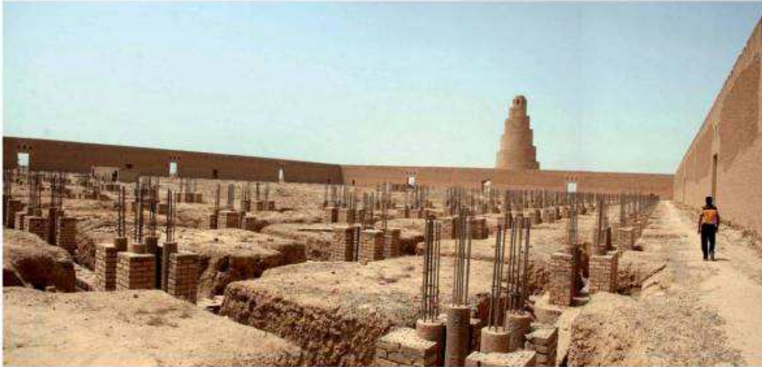
Foundation of the concrete columns reconstructed to roof the porticoes of the mosque.
