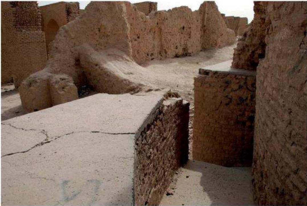
Cement protection of the wall minaret ramp, Abu Dulaf Mosque.
