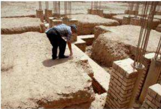
The concrete columns for the reconstruction of the portico.
