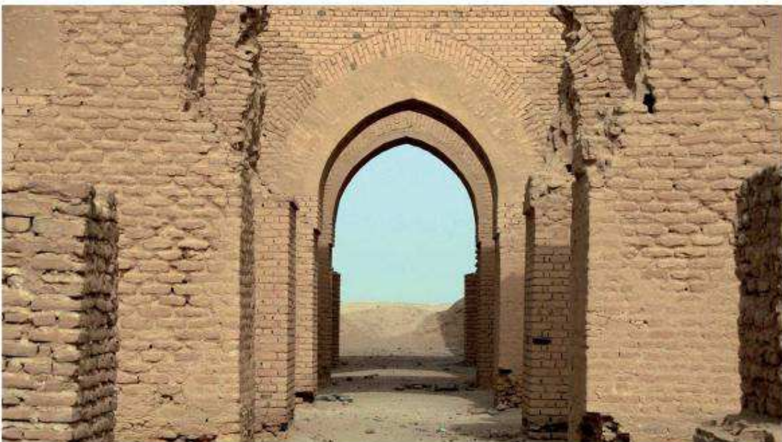
Basal erosion and reconstructed arches of Abu Dulaf Mosque.
