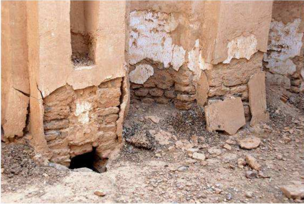
Wall base erosion due to humidity and salts.
