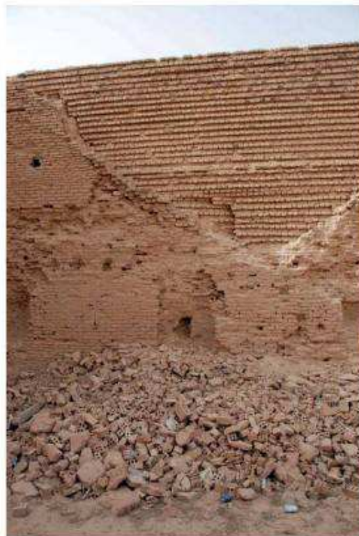
Erosion problems due to the incompatibility of materials, the reconstructed walls of the Al-Ma'shuq Palace.
