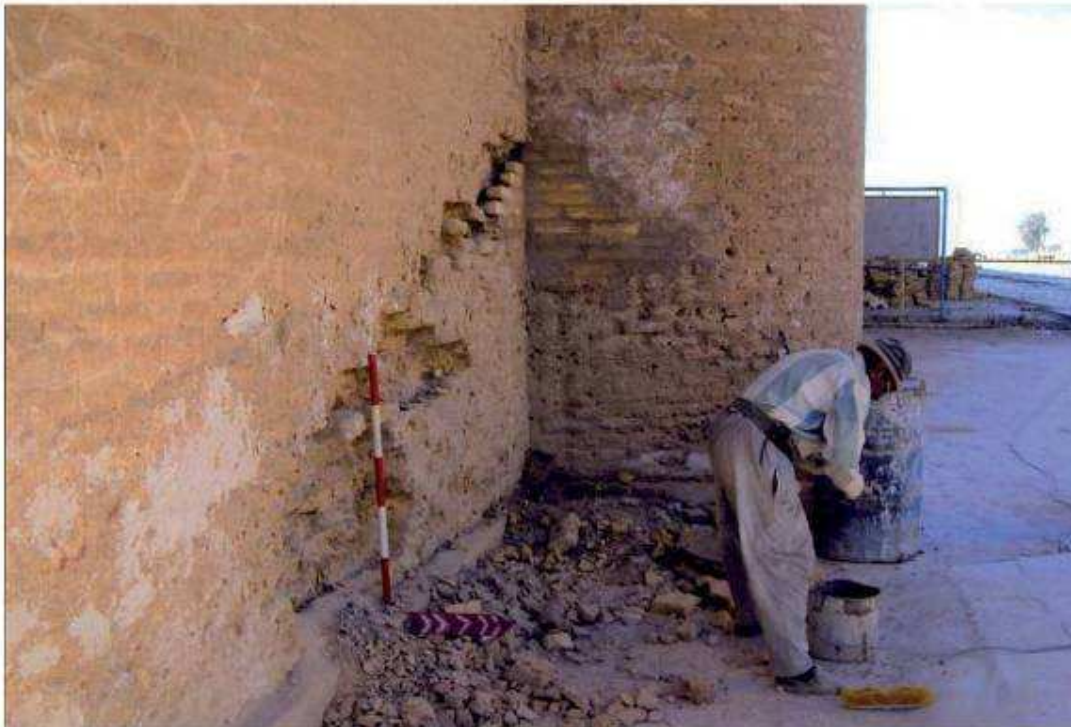
Treatment of basale erosion due to humidity and salts.
