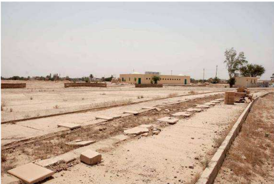
The intrusive concrete platform and cement pavement of the new walkway.
