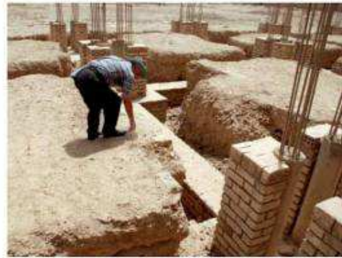
Foundation of the concrete columns reconstructed to roof the porticoes of the mosque.
