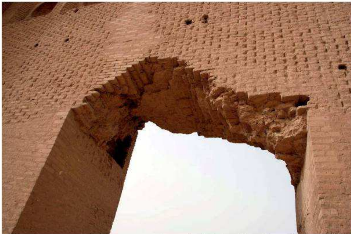
Structural pathologies, missing of the gate lintel, north façade.
