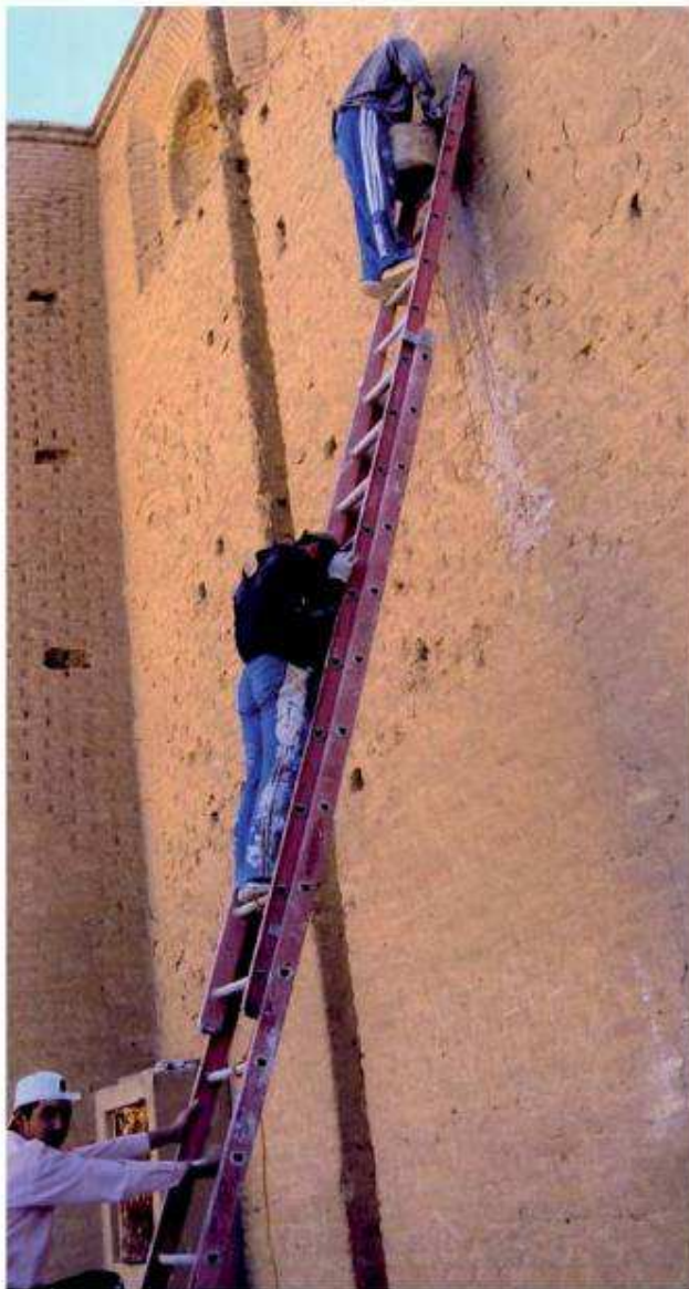
Great Mosque, vertical crack repair
