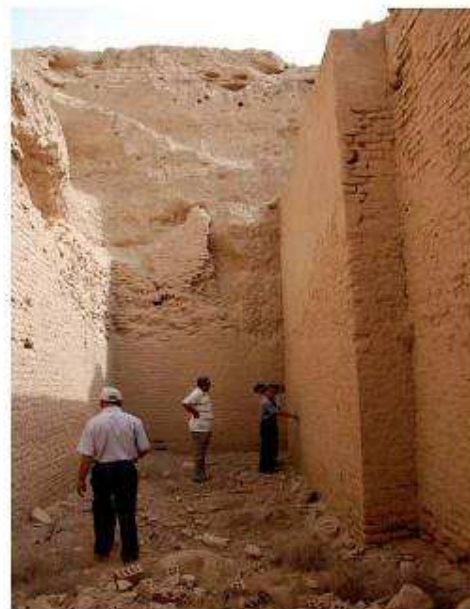
Poor quality of materials (modern fired bricks and concrete) used in the restoration of the Circular Basin.
