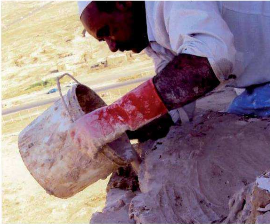
Use of traditional materials «Djuss» for the restoration works.
