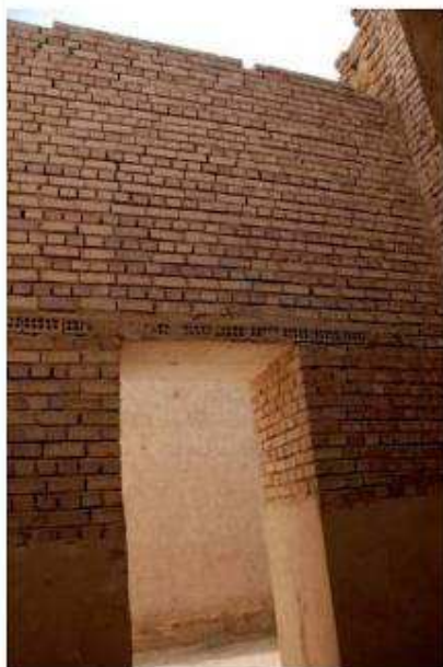
Poor quality of materials (modern fired bricks and concrete) used in the restoration of the Circular Basin.
