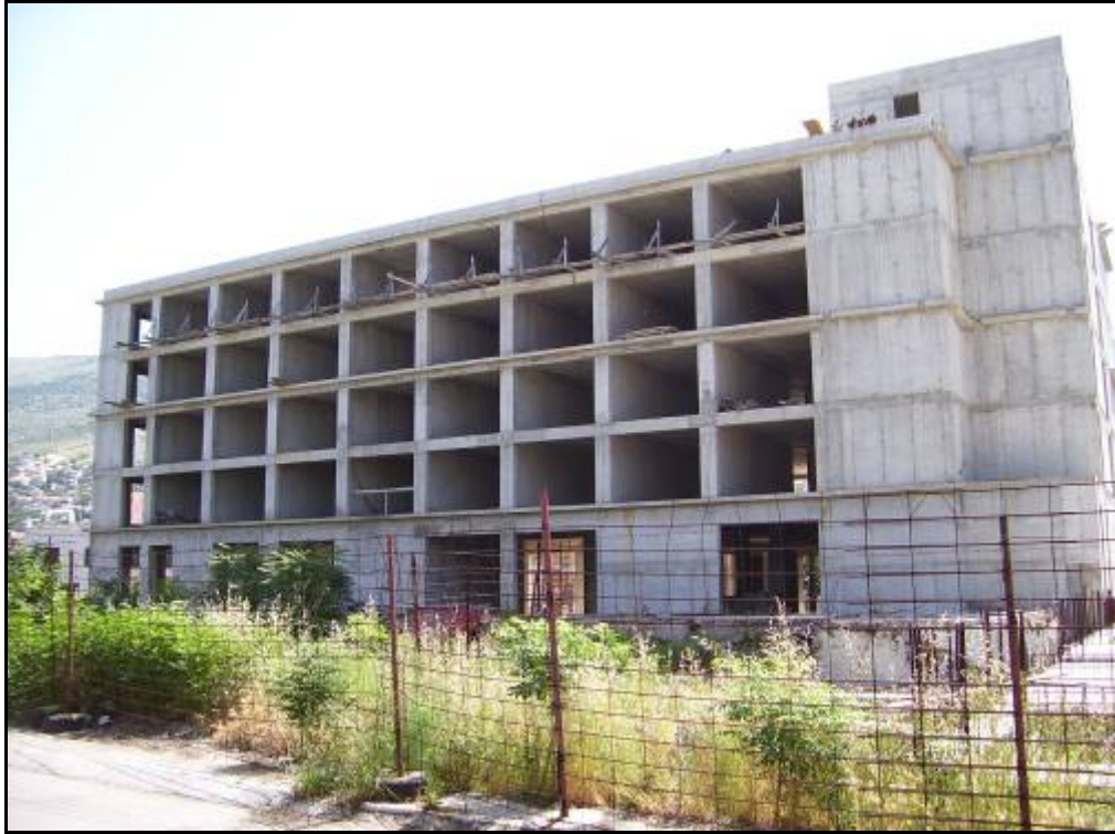
Front view of the building under construction
