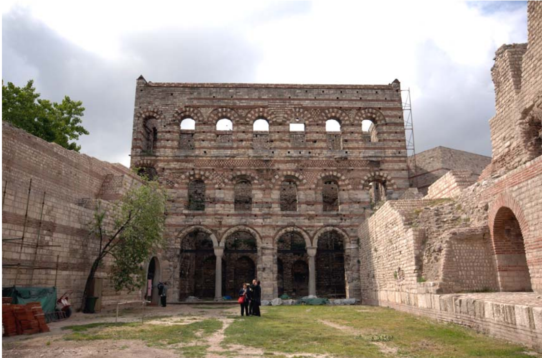
Above: Tekfur Saray, a Byzantine palace building. Work carried out to the adjacent walls since the 2006 mission involved excessive replacement of facing stones and bricks and the creation of new flat wall tops.
