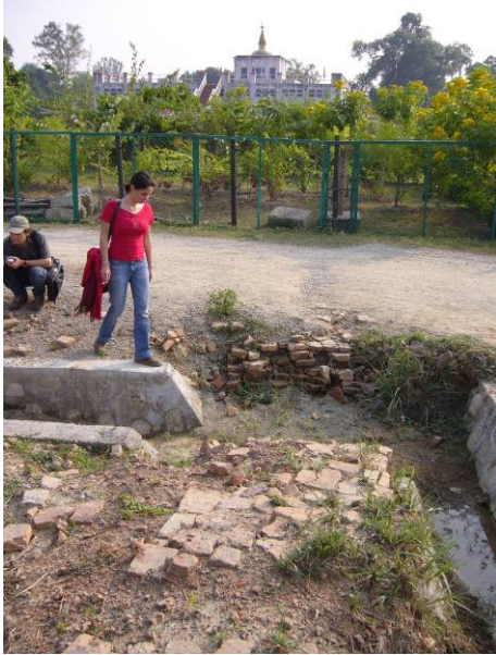
10. Important archaeological structures (a Vihara?) outside the core area were damaged by the digging of a drainage trench. The current boundaries of the WH core area must be reviewed
