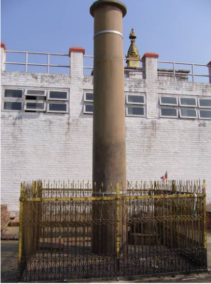
4. The visual and functional connection between the Maya Devi Temple and the Ashoka Pillar (see photo N.1) has been affected
