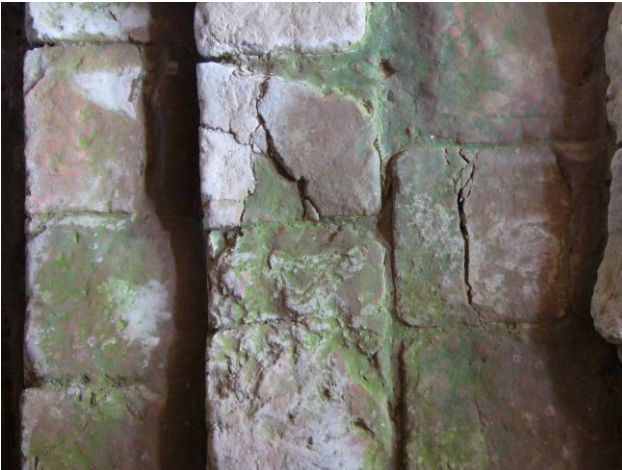
8. Moss and efflorescence from water in the ground
