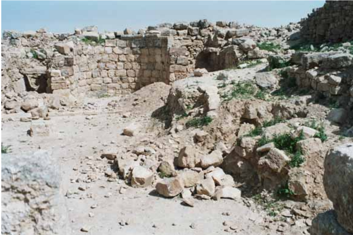
Fig. 17 - chaos left by recent collapses
