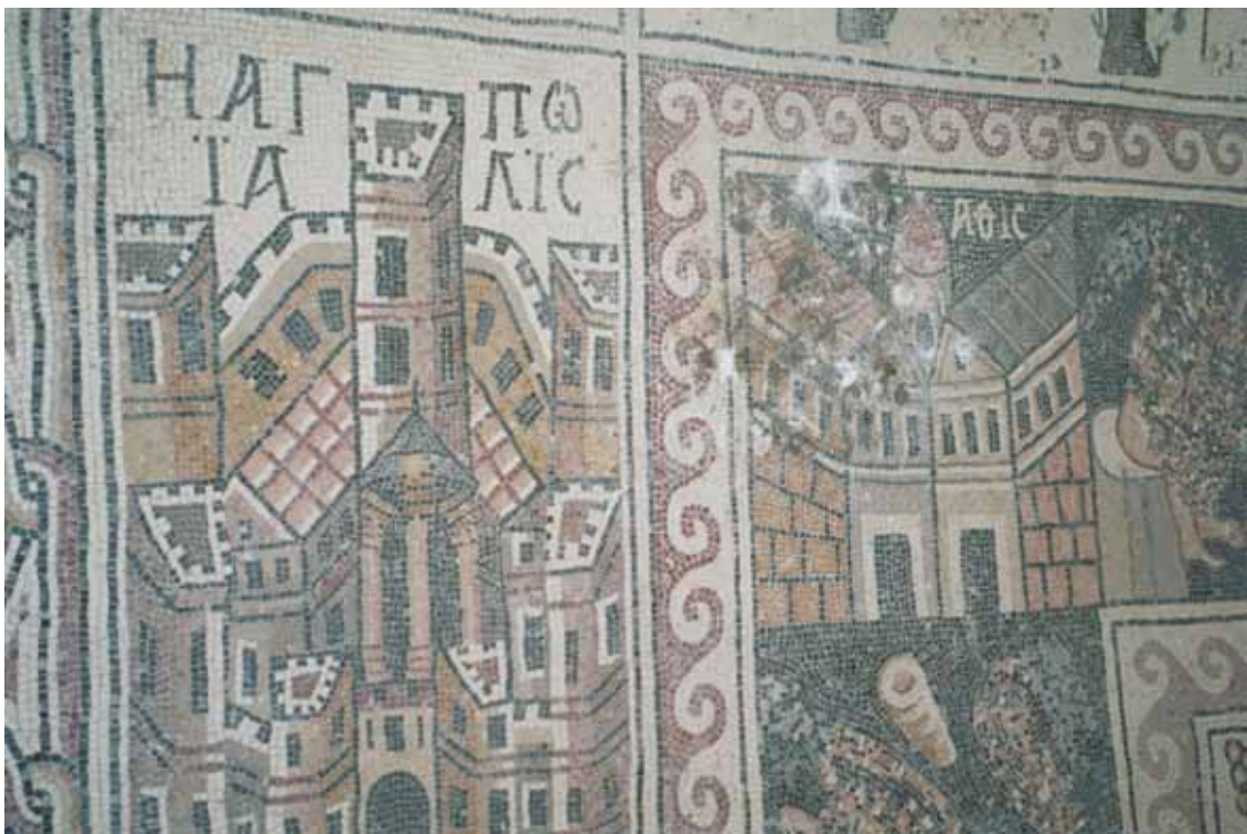
Fig. 27 – damage from humidity on mosaic floor of sheltered St. Stephen Church
