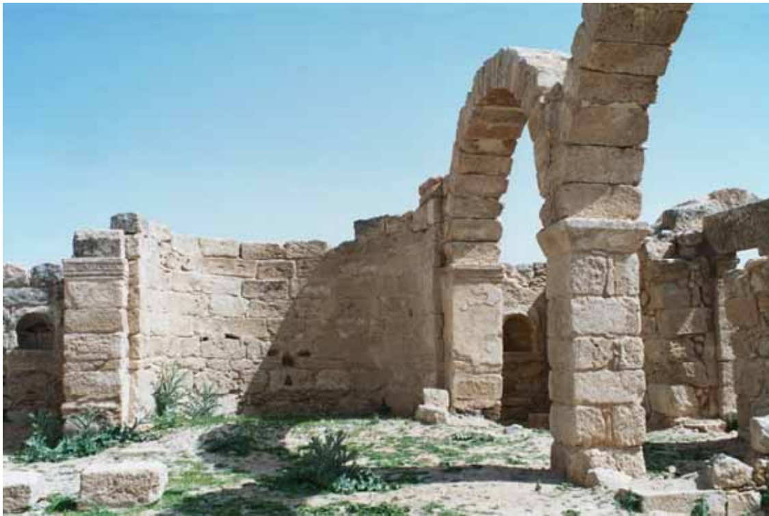
Fig. 16 – Shrubby vegetation grows on earth layer covering mosaics in S. Paul Church
