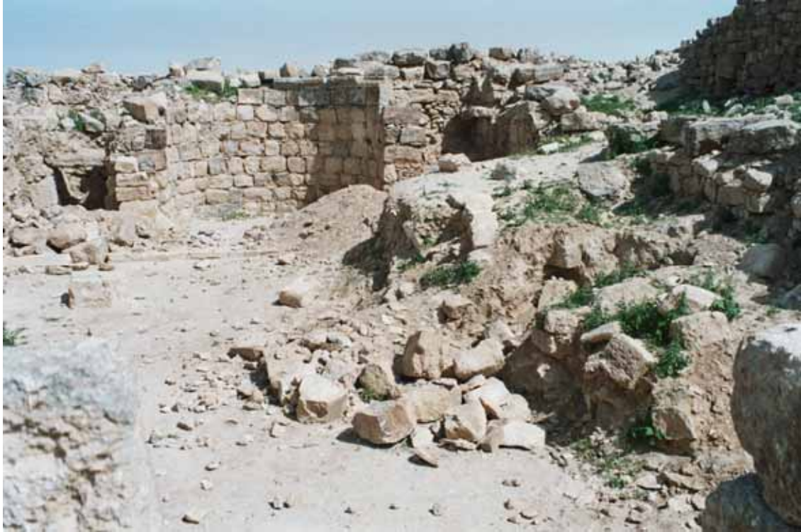
Fig. 7 – dangerous situation for visitors and structure
